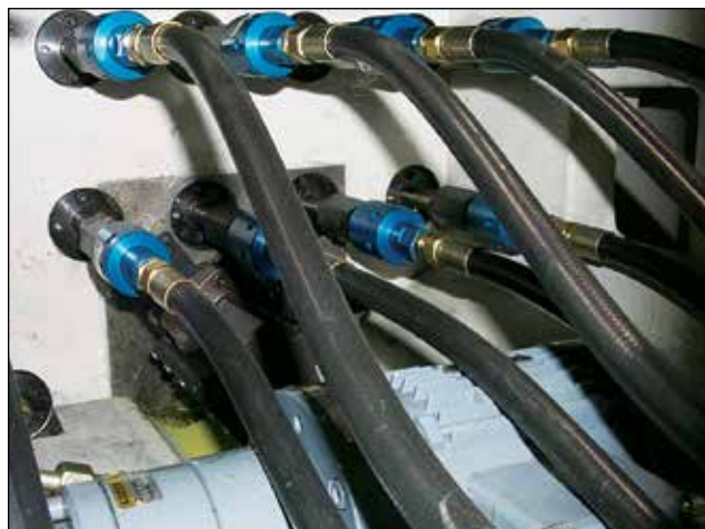
DEUBLIN 1116 Bearing-Supported Unions on Automotive Transfer Line
